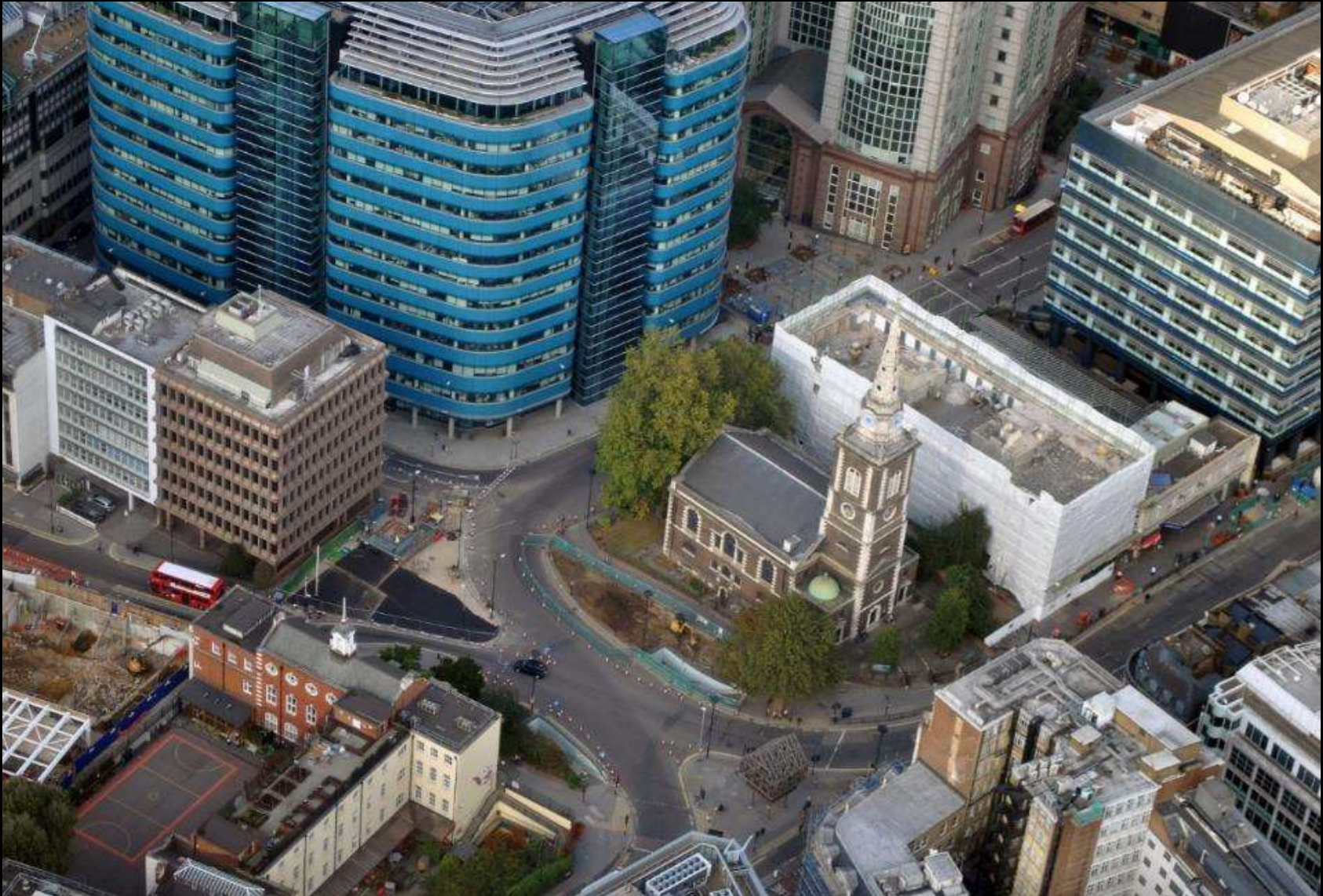
Aerial photograph of Aldgate Gyratory (before)
